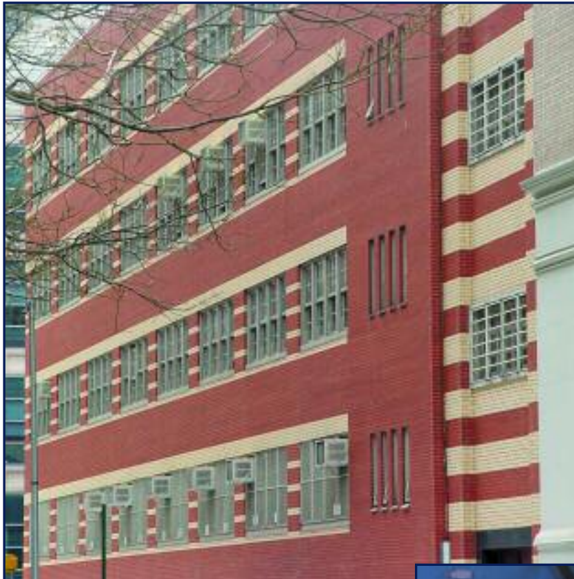
Above: Westinghouse High School, Downtown Brooklyn AM&G’s work included removal and reconstruction of the entire brick facade.
